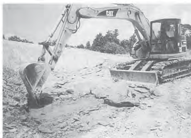
Fig. 4 The excavation site in August – September, 2000. The mud bed covering the shell bed (II) was removed by power shovel.
