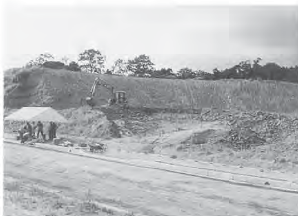
Fig. 5 The excavation site in September, 2000.
